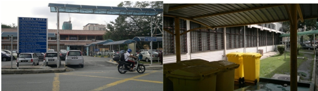
Figure 6: shows the façade of the main entrance of the two-storey building with the ground floor constructed with concrete to support the upper floor constructed with timber. The second picture shows the exterior window of the ward area with short overhang
