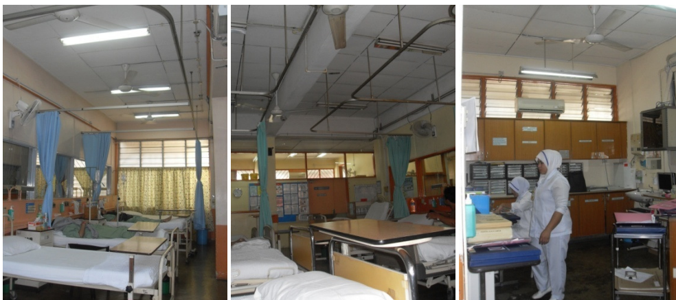
Figure 7: The interior view of ward area and nurse station. The windows availability are at one side of wall which close all the time with view of next building distance of 0.6 meter only. The nurse station's high cabinet almost cover the windows with no view
