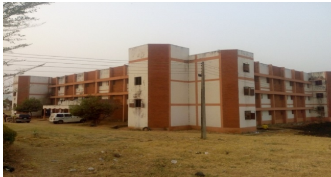
Figure 1: Front view of hostel Block A for male students at Gidan Kwano Campus
