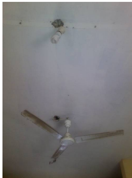
Figure 9: A room with ceiling fan
