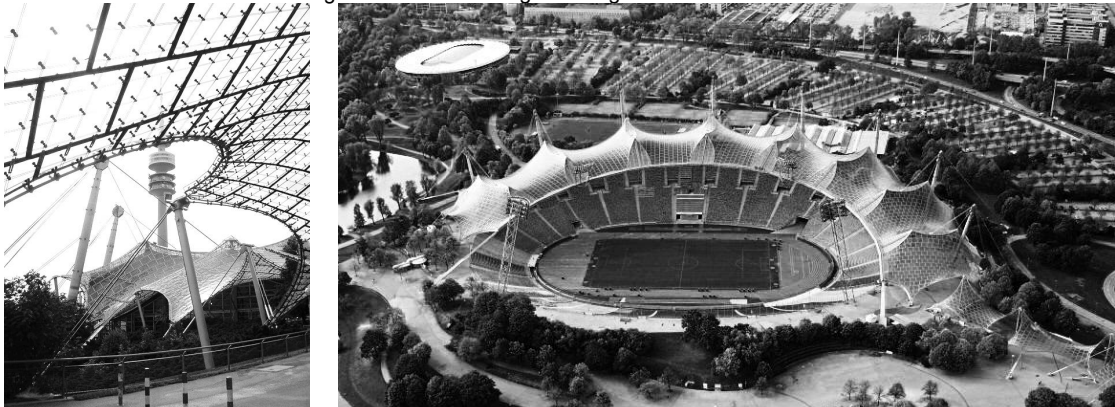
Figure 6 : Otto's designs in Olympic Stadium
