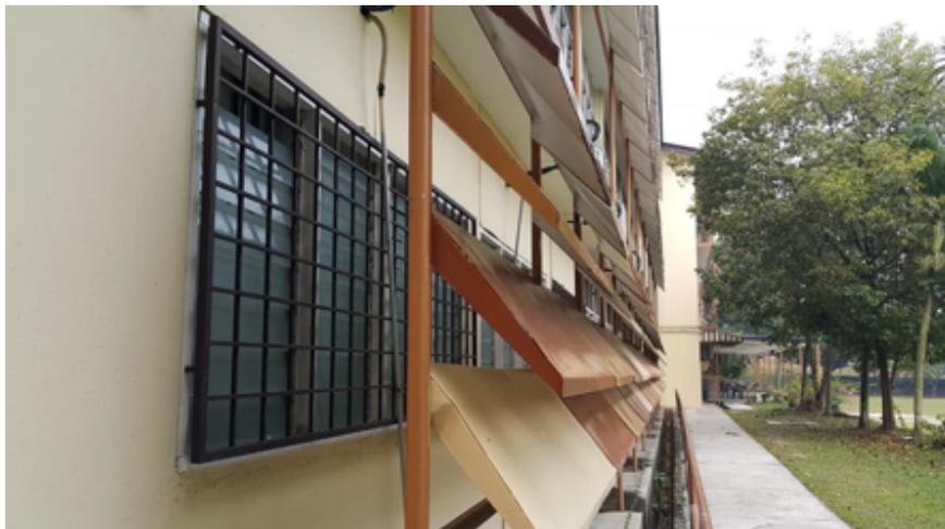
Figure 7: Shading device installed on the external side of the classroom of School A.
