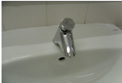
Figure 9: Self-closing tap (low flow tap)
