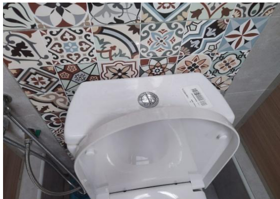
Figure 7: Dual flush use at building B
