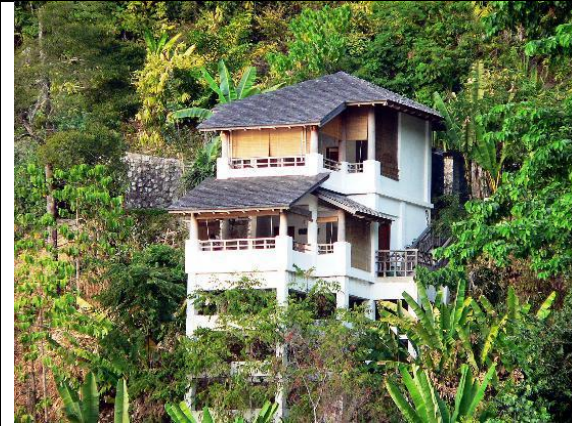
Figure 1: A chalet on the hazardous slope in The Datai Langkawi as the result of emphasising view towards the sea. Source: Author
