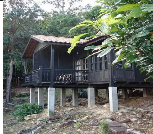
Figure 2: An example of chalet elevated on stilts at slope area implying the intention of preserving the environment. Source: Author
