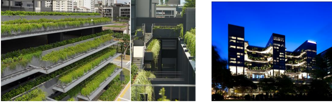
Teres langit di Skyterrace@Dawson dan Hotel ParkRoyal , Singapura (Sumber: http://www.scdarchitects.com/landscape/skyterracedawson , https://images.adsttc.com/media/images/5175/6287/b3fc/4b20/1400/012e/slideshow/PARKROYAL_2-2013_PBH_018.jpg?1413994925 Mac 2018 )
