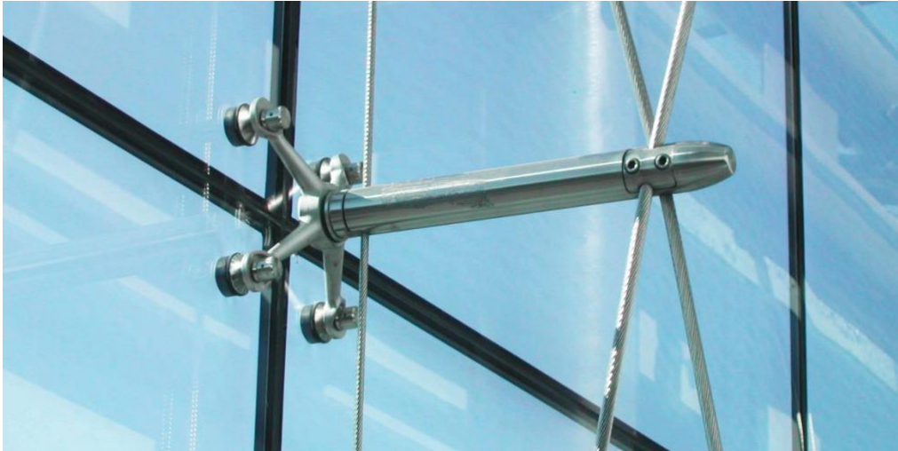
Gambarajah 4: Contoh "Glazing on Cable Truss" dalam rekabentuk bangunan. Harvard Medical Building: New Research Building (Sumber: https://enclos.com/project/harvard-medical-school-new-research-building/ )
