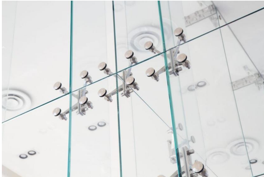
Gambarajah 2: Contoh “ point support glazing ” dalam rekabentuk bangunan. KIA Store Point Support Glass Façade - Ensanada, Mexico. (Sumber: https://www.cnmorn.com/kia-store-point-support-glass-facade.html )
