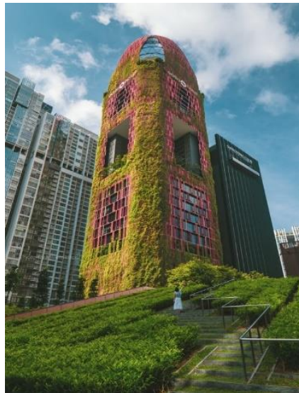
Rajah 1: Fasad hijau terus di Hotel Oasis Downtown, Singapura. Sumber: Designboom. 2019. WOHA's oasia hotel conceived as a living green tower in downtown Singapore. https://www.designboom.com/architecture/woha-oasia-hotel-downtown-singapore-living-tower-12-07-2016/ [12 Disember 2019].
