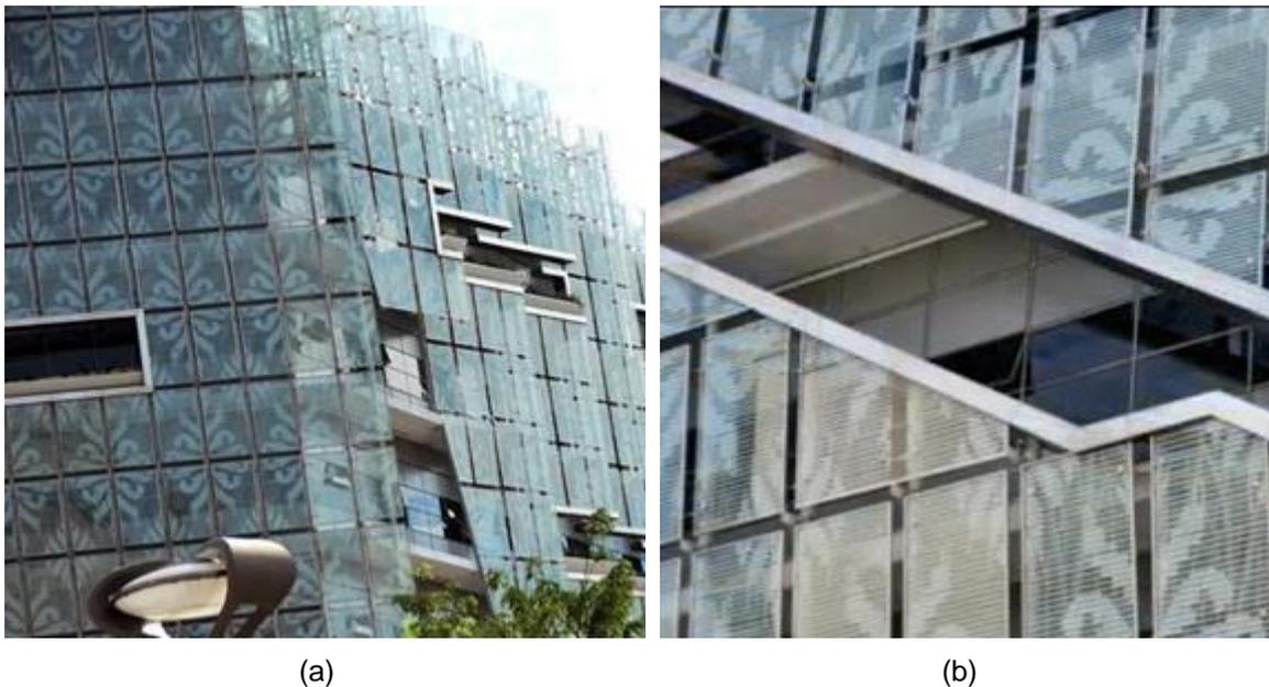
Figure 5. Pattern design that can be seen on the DSF at the Suasana PJH Building, Putrajaya. (a) View from the outside (b) Close up view (Otodesign, 2022).
