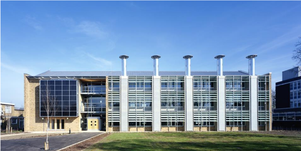
Figure 7: Front View of Building Research Establishment, United Kingdom.
