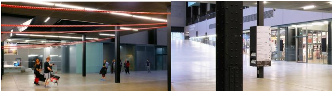
Figure 16: The creative lighting strategy for Tate Modern had to provide daylight and electric lighting to create a high-quality lit environment for visitors internally with the usage of previous the steel structure from the old power station until nowadays
