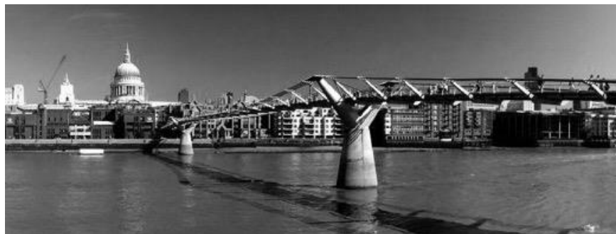
Figure 3: The millennium bridge completed in 2000 and reopened in 2002 after the wobbly occurrence
