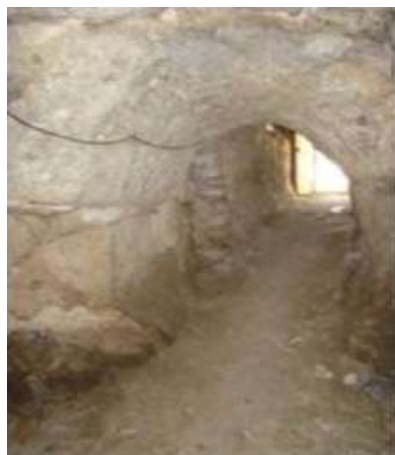
Figure 7- Entrance from inside .
